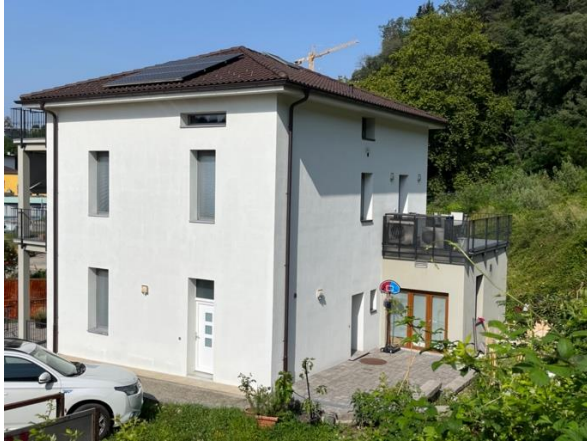
Figure 11: Outdoor unit on the balcony
