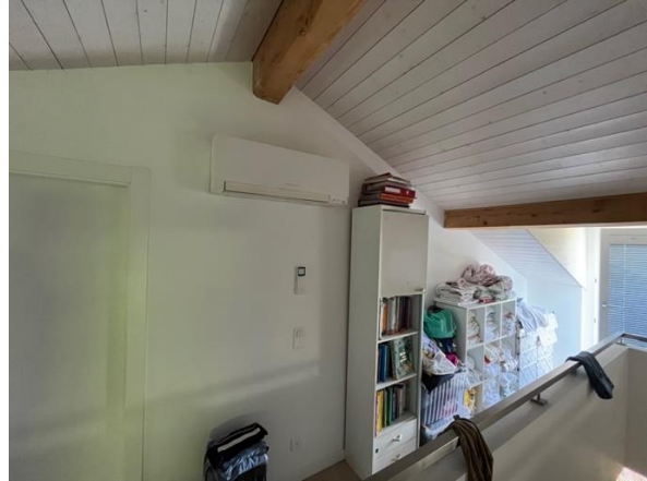
Figure 12: Interior unit in the studio below the roof
