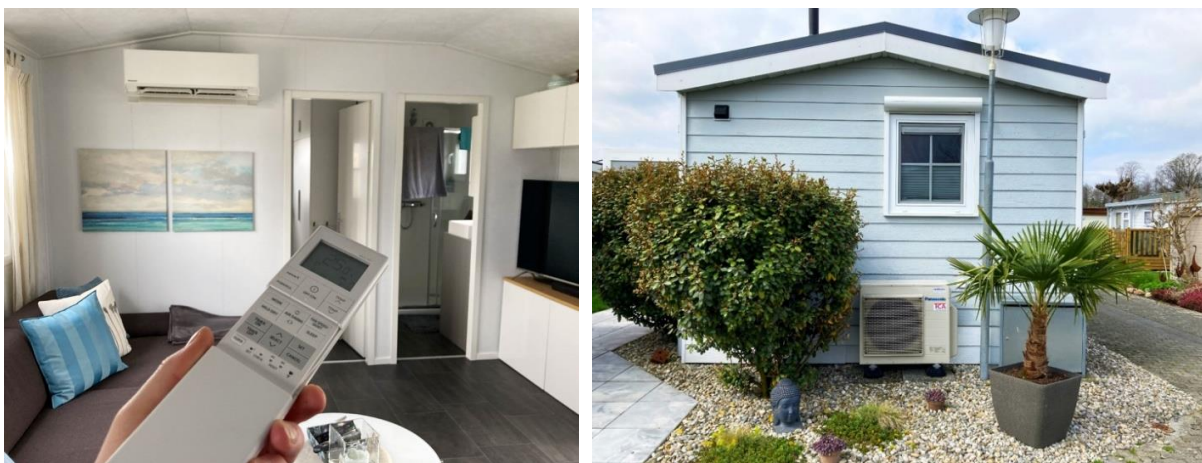
Figure 6: This mobile home is heated with an outdoor unit and 3 indoor units by Panasonic.
