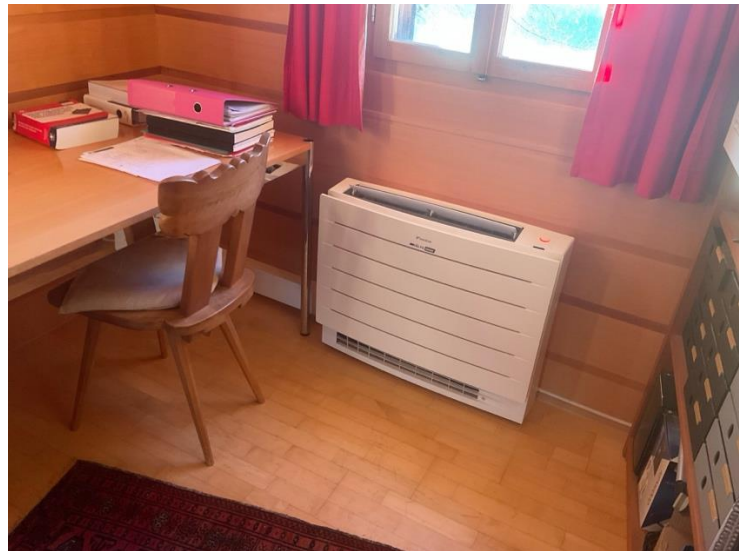
Figure 10: Internal unit of the AC
