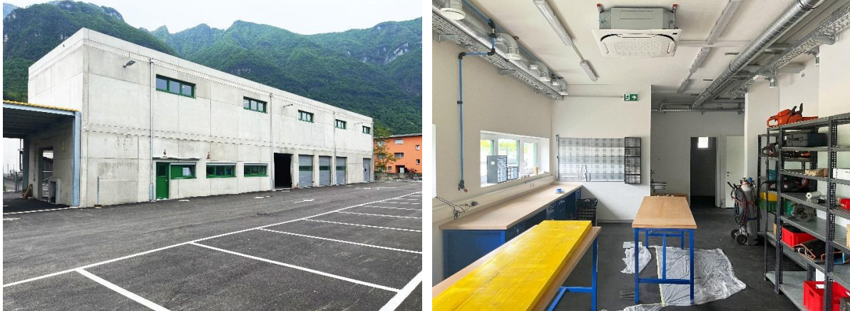
Figure 7: Recycling centre with municipal depot (with high energy efficiency standard). The office, reception, repair workshop, cloakrooms and the sanitary facilities (showers and toilets) for the employees are equipped with a VRF system by Daikin.
