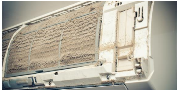
Figure 20: Dusty filters of an inside unit
