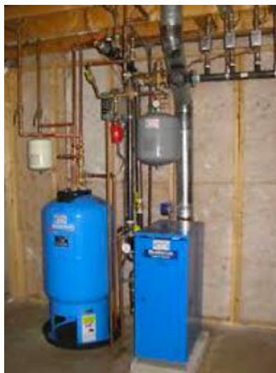
Figure 3: Example of gas-fired boiler
