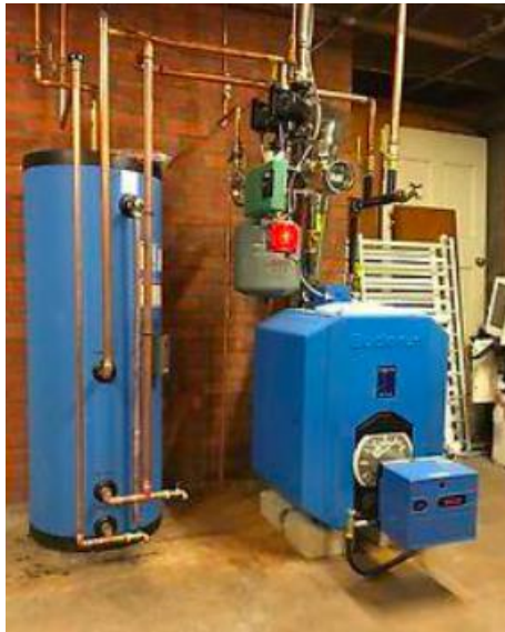
Figure 2: Example of an oil-fired boiler
