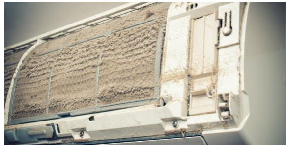
Figure 20: Dusty filters of an inside unit
