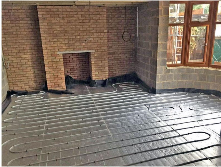
Figure 1: Installation of an underfloor heating pipes
