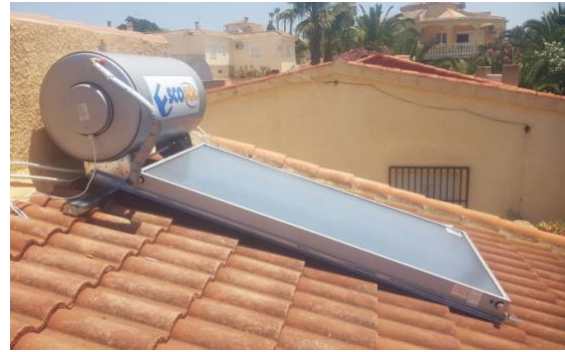
Figure 13: Example of an installed solar assisted electric storage water heater
