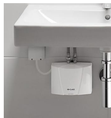
Figure 3: Schematic representation of an electric instantaneous water heater
